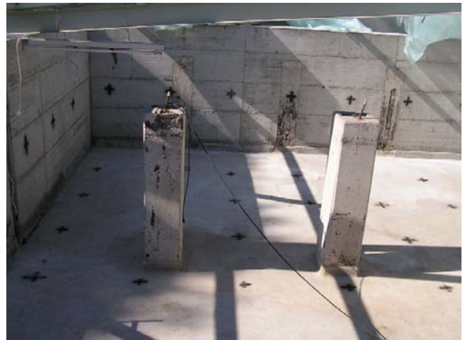
Fig. 2: Grid areas used in clearing the controlled area at Lucens.
