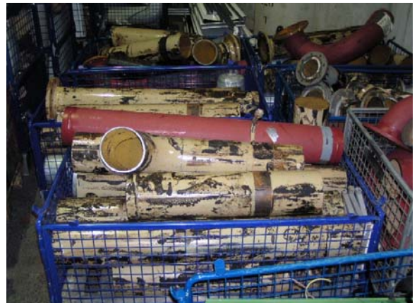
Fig. 3: Cleared cooling piping at KKM
